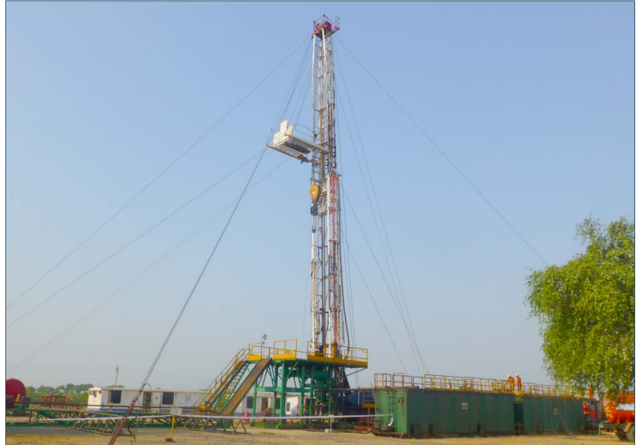
Workover rig at Cambay-19z
