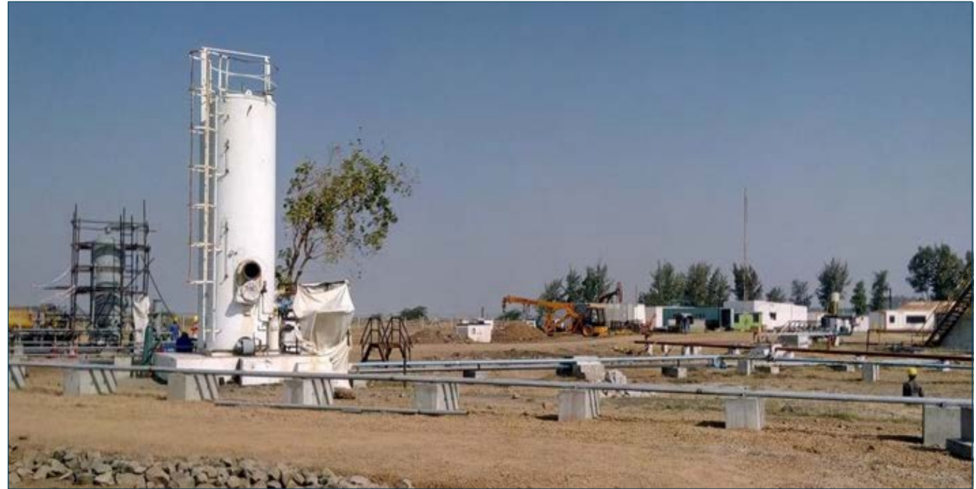
Bhandut early production facility construction
